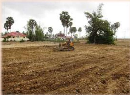
Fill was required to raise the level of the site above wet season water levels. This was extracted from one section of the CLS land and spread on the adjacent section where the playing field oval was to be constructed.
