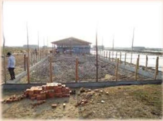
Construction started in April 2015 with filling of the site to raise it above wet season flood levels. Containing walls were built and sand was imported to provide a soft playing surface. A high fence was erected to enclose the oval.
